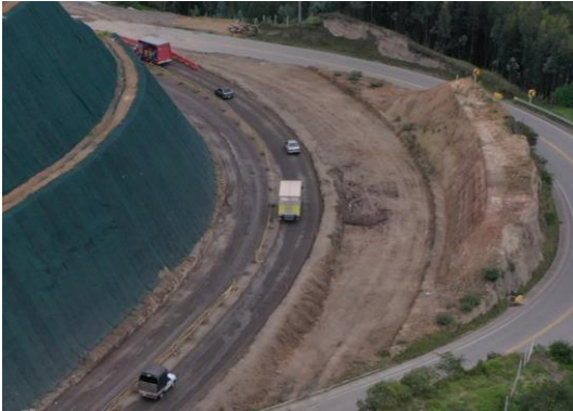
PL124 Sub base granular
